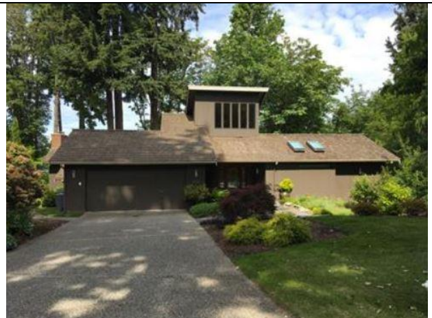
Plate 1. East (Lake side) view of the house, looking west from Forest Avenue SE.
